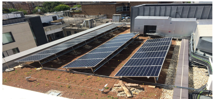
Roof area 15 - ABG bluerooF with biodiverse & PV finish
