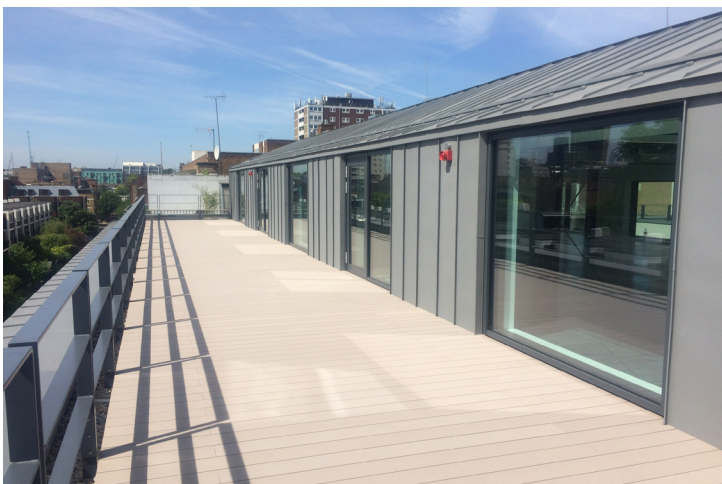
Roof area 9 - ABG bluerooF with decking surface finish
