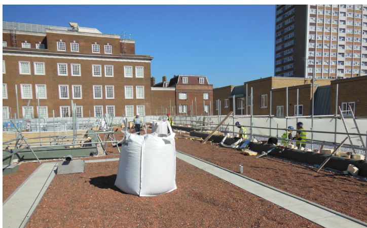
Pathways installed to make the roof accessible to all
