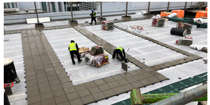
Installing paved finish to Level 60
