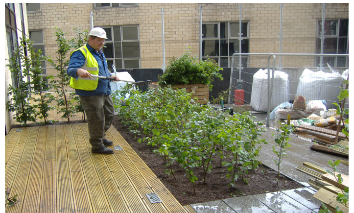
Final planting installation
