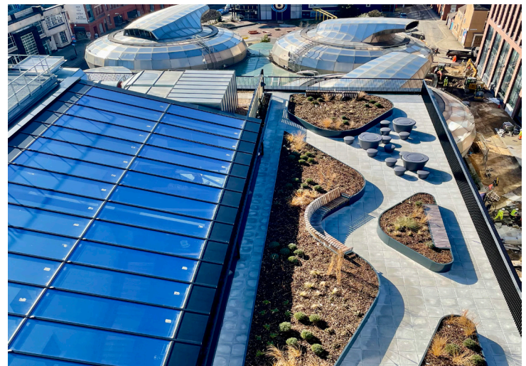
Langsett Building rooftop (Block D) on Howard Street
