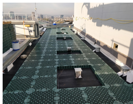
Void formers being installed to roof level 10
