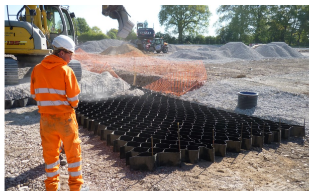
Fig. 8: Abweb fully pinned into position
