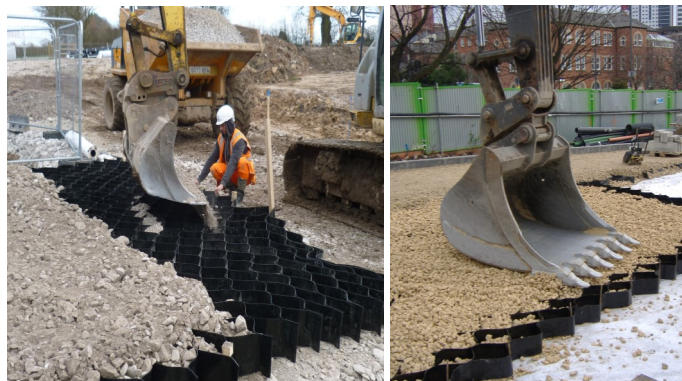
Fig. 11: Abwebs being backfilled & compacted
