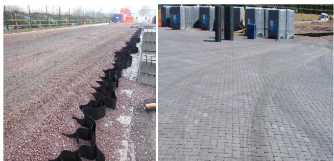
Fig. 12: Example of Abweb as base layer for final surface
