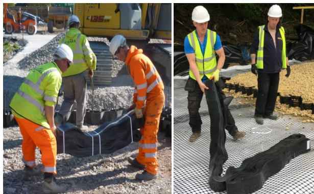
Fig. 6: Carrying & uncoiling Abweb into place
