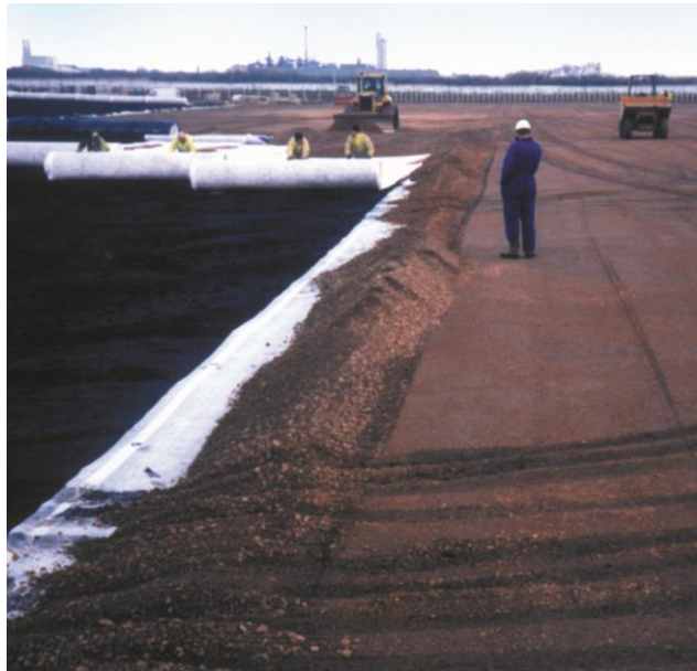
Large rolls enabled rapid installation
