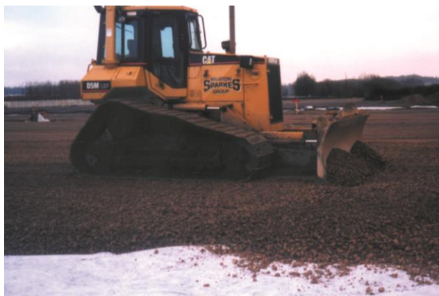
Plant operating on 150mm of Type 1 backfill material
