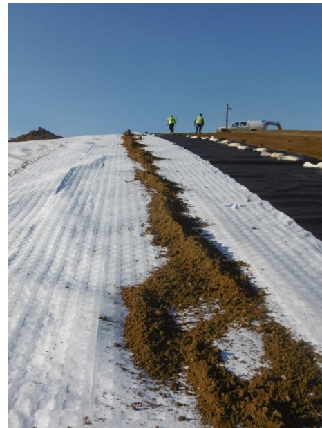
Figure 5: Landfill cap construction
