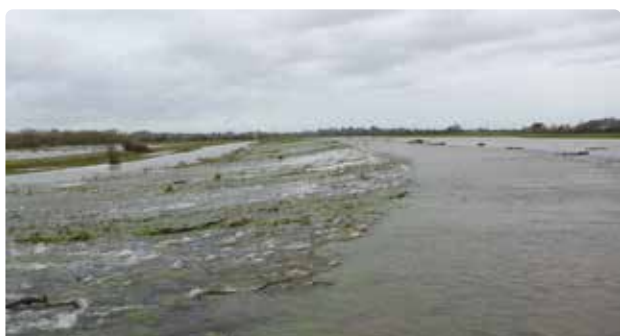
Aller Moor reinforced grass spillway, Somerset Levels Erosamat Type 3/20Z permanent reinforcement for flow velocities up to 7 m/s (vegetated)
