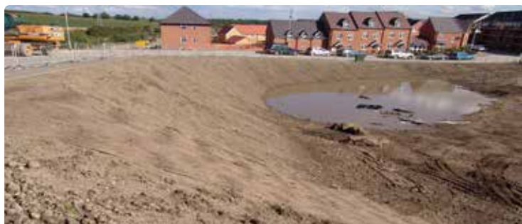
Barratt Homes Development, East Ardsley, Leeds Erosamat Type 1 for surface erosion control
