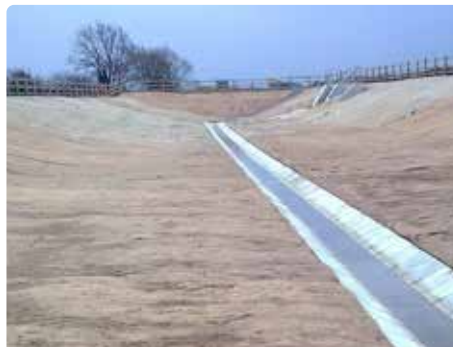
Leeds Bradford Airport, SuDS basin Erosamat Type 4K for surface erosion control
