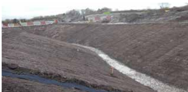
Henthorn Road housing development, Clitheroe Erosamat Type 3/20Z permanent reinforcement for drainage channel
