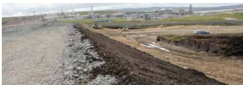
Sullom Voe Gas Terminal, Laggan-Tormore Roadbridge, Shetland Islands Erosaweb panels for embankment stability and topsoil containment
