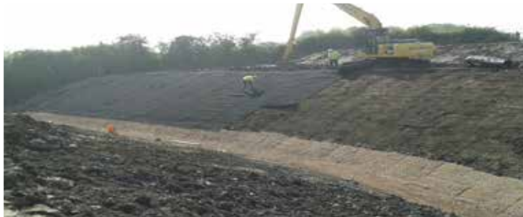
Henthorn Road housing development, Clitheroe Erosamat Type 3/20Z permanent reinforcement for drainage channel
