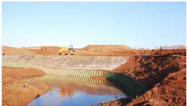
Bellway Homes development, Calverton Road, Nottingham Erosamat Type 1 for temporary soil cover on cut slope above ABG Webwall retaining wall
