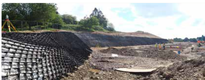
University of Exeter, East Park student accommodation Erosaweb panels for topsoil containment above stone faced soil nail retaining wall
