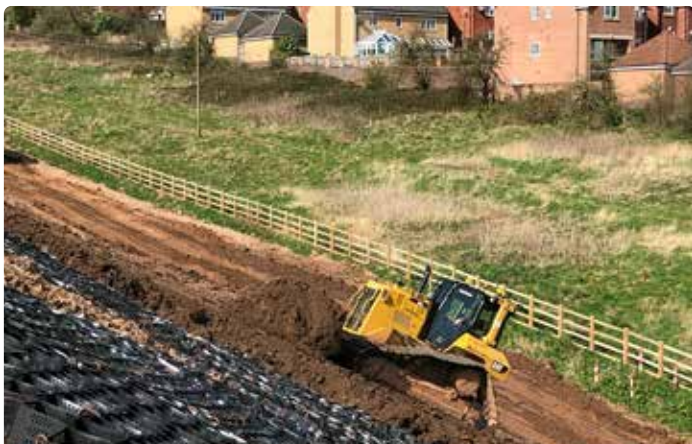
Gedling Access Road, Nottingham Soil containment for 1:2 slope to maximise adjacent flat land for development
