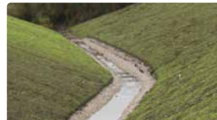
Leeds Bradford Airport, SuDS basin Erosamat Type 4K with vegetation established
