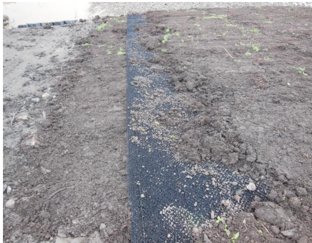
Erosamat's open three dimensional structure allows the product to quickly bind with root systems
