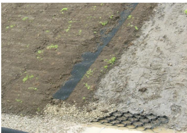
Erosamat (slope) & Erosaweb (base) used in combination to form a complete geosynthetic solution
