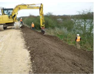
Topsoil is placed on the slope, overlain with Erosamat, pinned into place and secured by an anchor trench at the top and bottom of the slope. it is then seeded and buried with a thin layer of additional topsoil.
