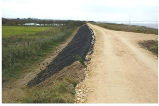
The Erosamat and anchor trench is ready for backfilled with topsoil. ABG Abgrid biaxial geogrid was used to reinforce the crest which acted as an access road.
