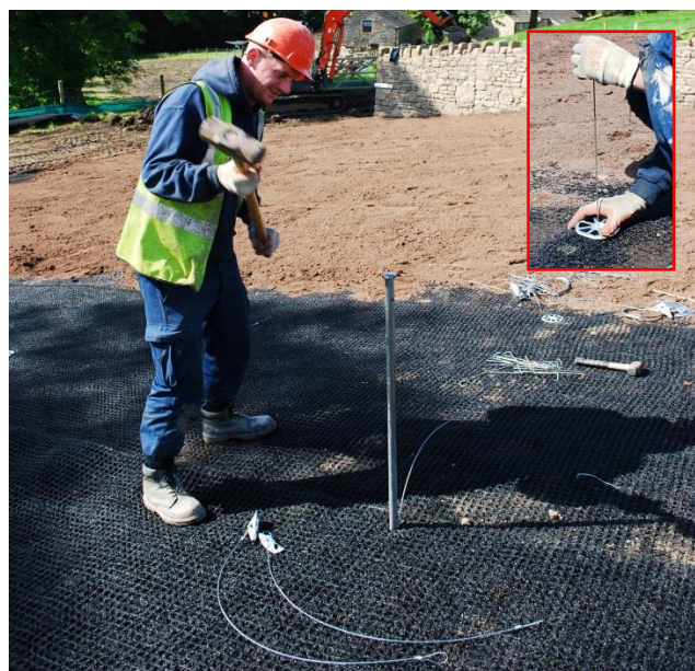
Ground anchors driven through soil. Washer placed over cable and tensioned against the geogrid.
