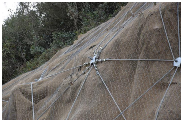
Erosamat adapts to the contours of the slope
