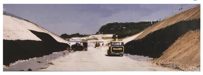
**Erosamat**'s three-dimensional open matrix was utilised to protect the less steep upper slopes from erosion and to provide permanent root zone reinforcement for the vegetation. 150mm of topsoil was placed on the chalk with the 20mm thick **Erosamat** pinned on top. The topsoil was hydro seeded with a drought resistant
