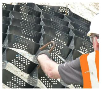
Steep, dry, barren chalk face covered with Erosaweb held with "J" pins ready to receive 150mm topsoil
