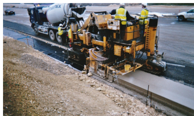
Fig. 9: Casting extruded channel overview
