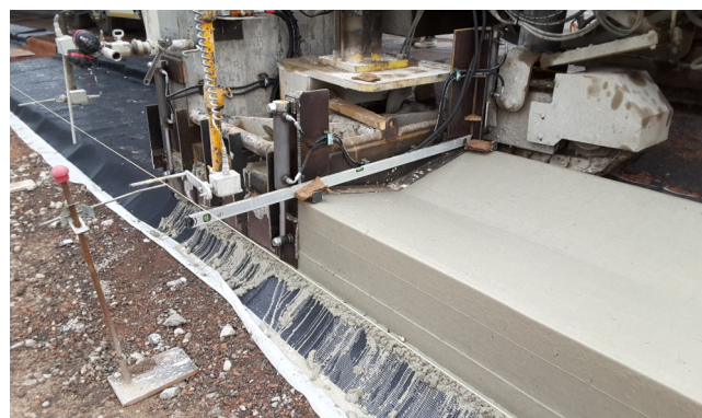
Fig. 8: Casting extruded channel detailed view
