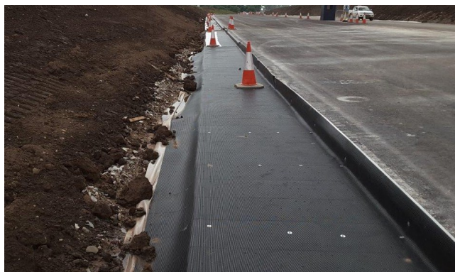
Fig. 6: Uprand nailed to base layer
