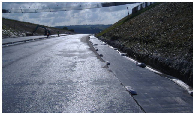
Fig. 5: Fildrain held down by sand bags to prevent wind uplift
