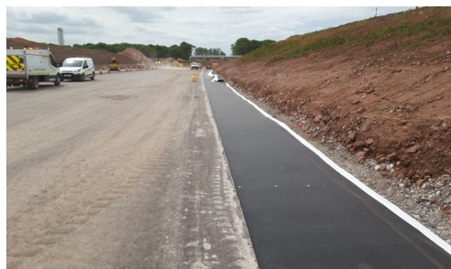
Fig. 7: Fildrain installed and ready for extruded channel
