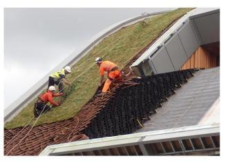
Installation of the geocellular system (Erosaweb) to retain growing media on slopes. All Geogreen operatives were Irata level 3 & 4 trained as rope access was critical.
