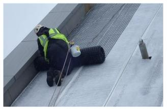
Reinforcement geogrid (Trigrid) secured to anchor points installed above the reservoir & drainage layer (Roofdrain).
