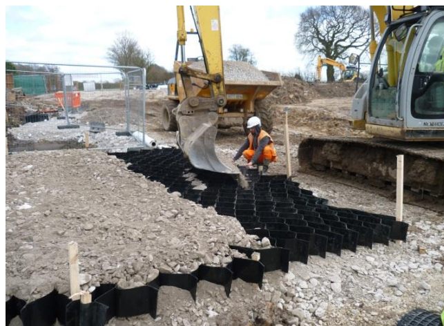
Abweb can provide a 50% reduction in the required thickness of sub-base
