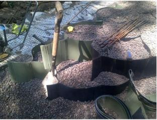
Webwall pinned into place in layers filled with the light-weight aggregate and compacted by hand. This created a stable reinforced retaining structure supporting the road with minimal load on the embankment.
