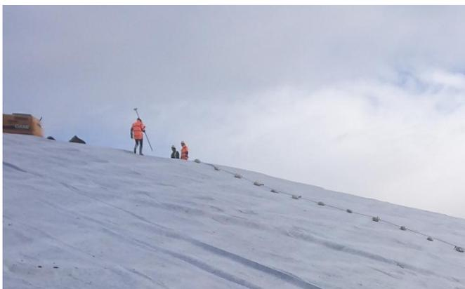
**Pozidrain is stable on steep slopes of up to 1:2.5 (21.8%)**
