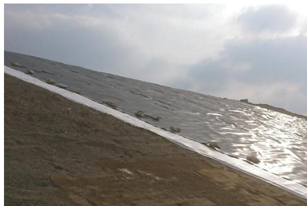
**Long, wide rolls enabled fast installation**
