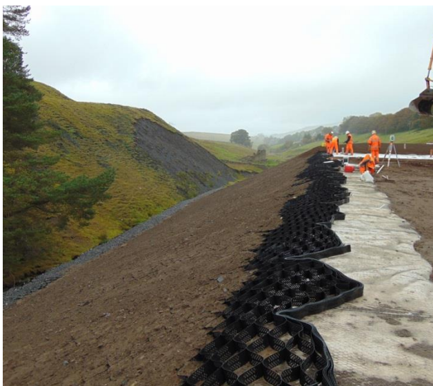
Erosaweb panels providing soil veneer reinforcement
