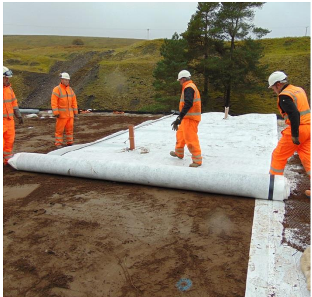
Wide width rolls enabled rapid installation and minimised the number of joints
