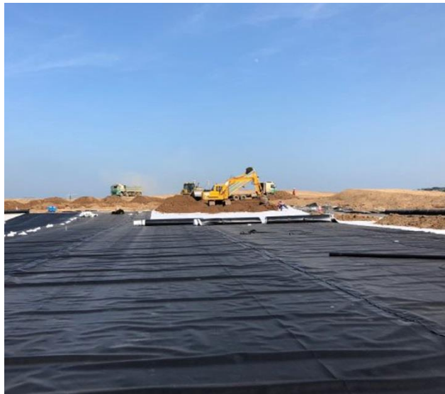
Large Pozidrain geocomposite rolls enabled rapid installation and superior drainage performance
