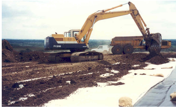
Fig. 13: Placing cover soil
