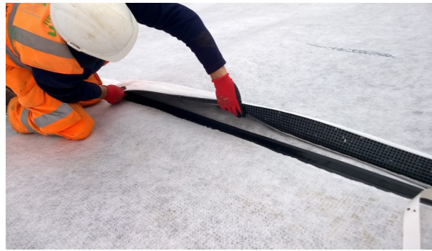
Fig. 8: Pozidrain K [L] Butt Joint with Butyl Tape
