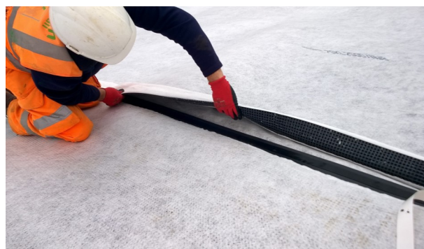
Fig. 9: Pozidrain K [L, H80] Butt Joint with Butyl Tape
