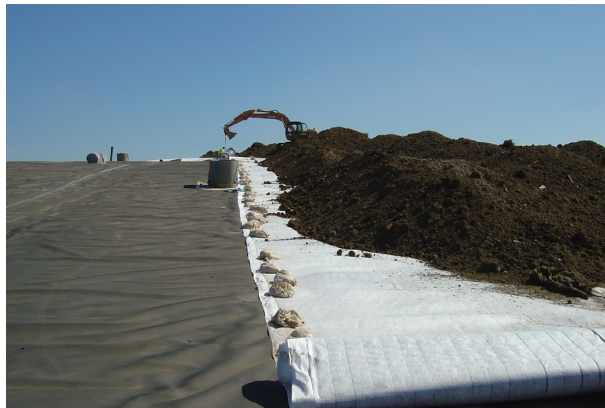
Fig. 6: Pozidrain K placed on steep slope
