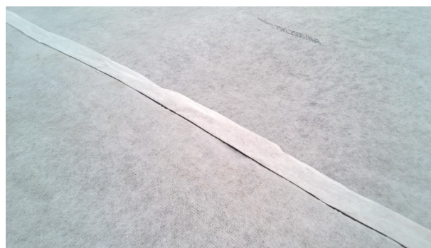
Fig. 10: Geotextile flap overlap
