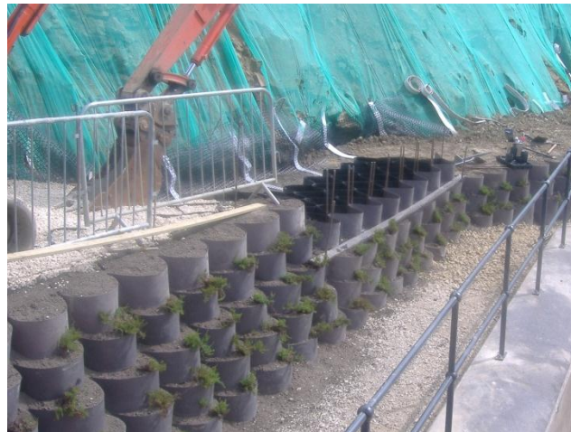
Webwall being constructed and filled
