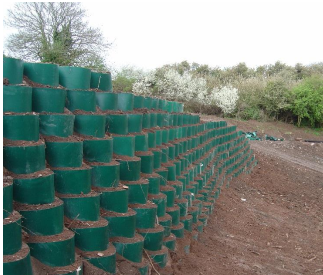
The green front face Webwall cells were seeded with a local wild flower mix
