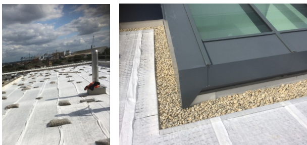
Fig. 10: Roofdrain cut around penetrations (e.g. vent chimney & roof light).
