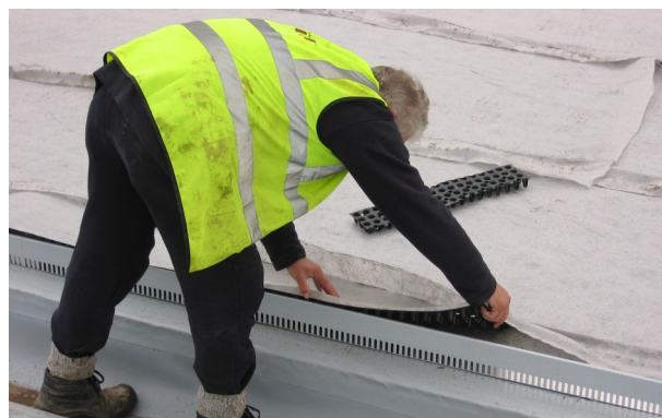
Fig. 13: Replacing a section of damaged core.
