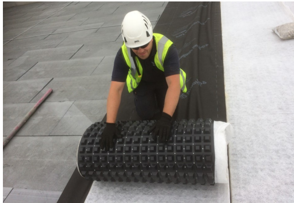
Fig. 5: Lay with geotextile filter & cuspat openings facing up.
