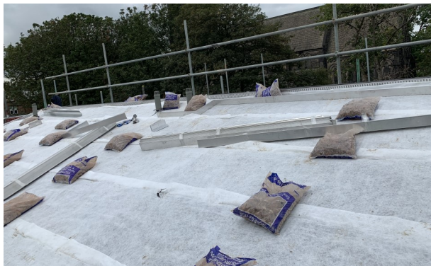
Fig. 8: Roofdrain installed to gently sloping roof, anchored at the apex.
