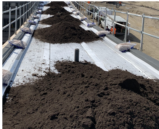
Fig. 12: Backfill with growing media (planted areas) or sand (paved areas).
