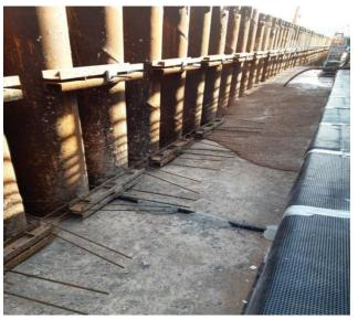
Concrete pour behind CHS pile wall. Deckdrain fixed to existing wall to channel surface & ground water from behind the new wall & promenade structure
