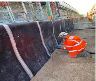
Deckdrain fixed to existing sea wall using Abfix pins & washers to maintain impermeability and jointing tape to prevent concrete ingress
