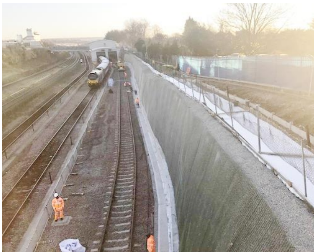
Finished retaining structure. The system using Deckdrain gained Network Rail engineer approval after trial
