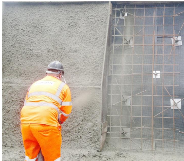
Installation trials demonstrated excellent adhesion of the sprayed concrete to Deckdrain
