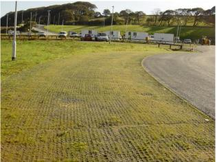
ABG Sudspave 40 is clipped together to create a continuous permeable reinforced surface. It is cut to fit the curving shape of the car park which fits the existing contours of the valley site. The high strength plastic supports the load of cars whilst allowing grass to establish quickly resulting in an aesthetically pleasing finish.
