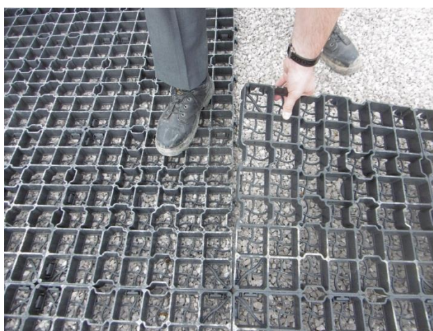
Easy to connect units with positive lug and slot.
