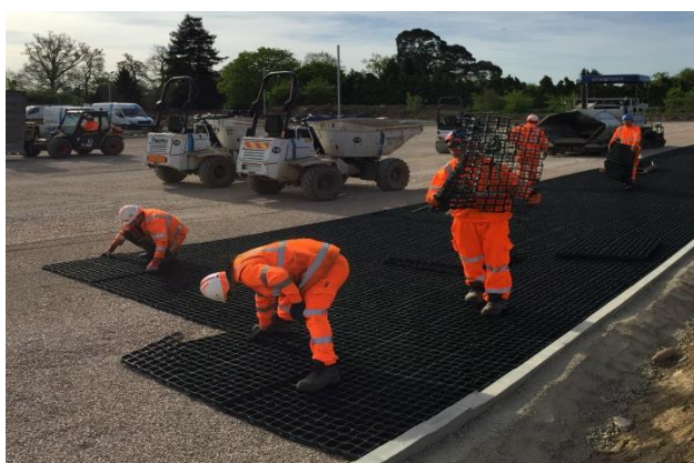
Installation of Sudspave made faster by pre-assembled panels
