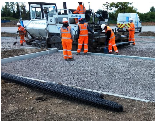
Installation of Abgrid stabilised sub-base and bedding layer
