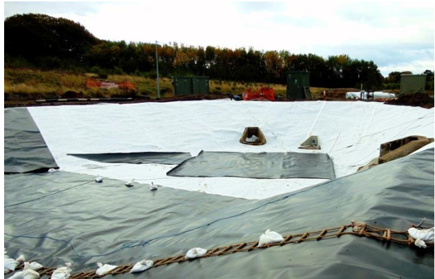
Pozidrain under the liner provides drainage, gas venting and puncture protection
