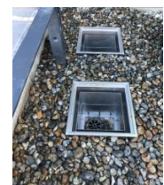
The blue roof restrictor chambers
