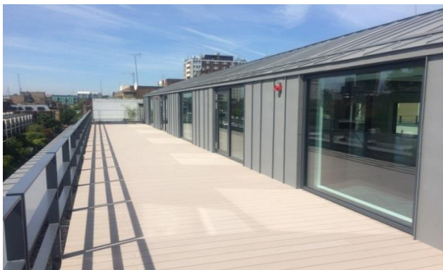
Roof area 9 - ABG bluroof with decking surface finish
