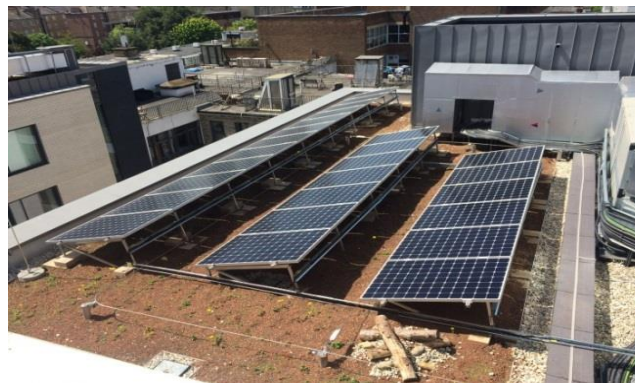
Roof area 15 - ABG bluroof with biodiverse & PV finish
