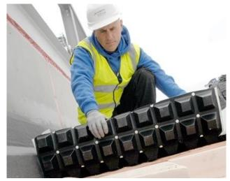
Placing the ABG green roof boards showing the overflow holes which then feed into the blueroof attenuation system below
